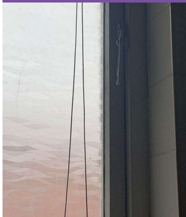
04-04-2022 11:59 / Bathroom Windows Sills / Kc6s6vq5l
