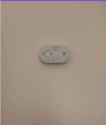
Expires 22-02-2023 in the utility room where boiler is kept.
