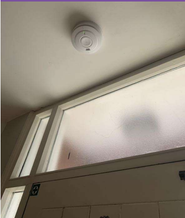
In the hallway by the front door expires 1-1-2027
