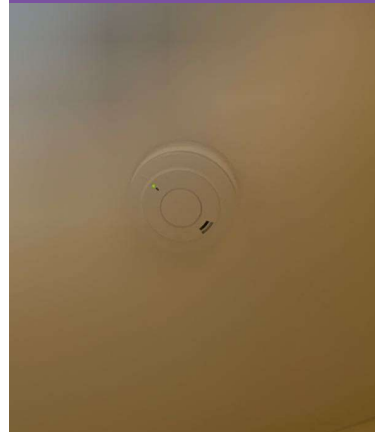
In the hallway at the top of stairs - expires 1-1-2027.
