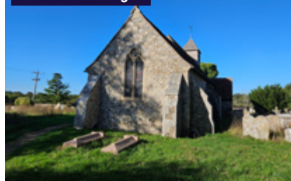
Work at St Mary's church Binsted has begun.
